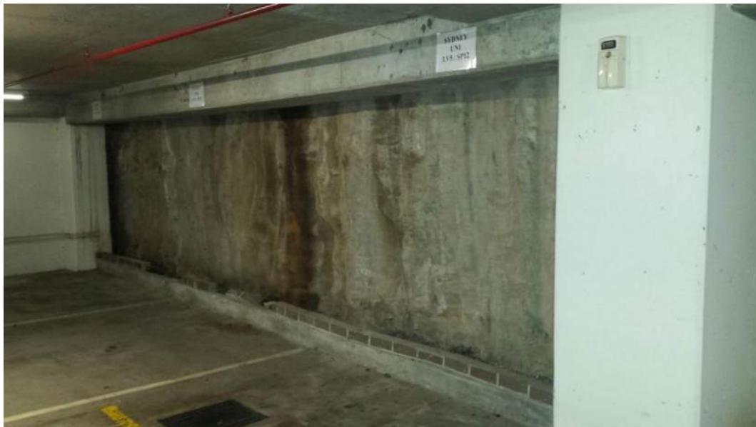
Figure 7: Level B5 Pitt Street boundary excavation
